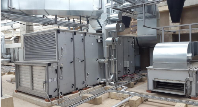
Fig. 3(b): Systemair Danvent DV 100 Fresh Air Handling Unit with Heat Recovery Wheels and Plug Fans
