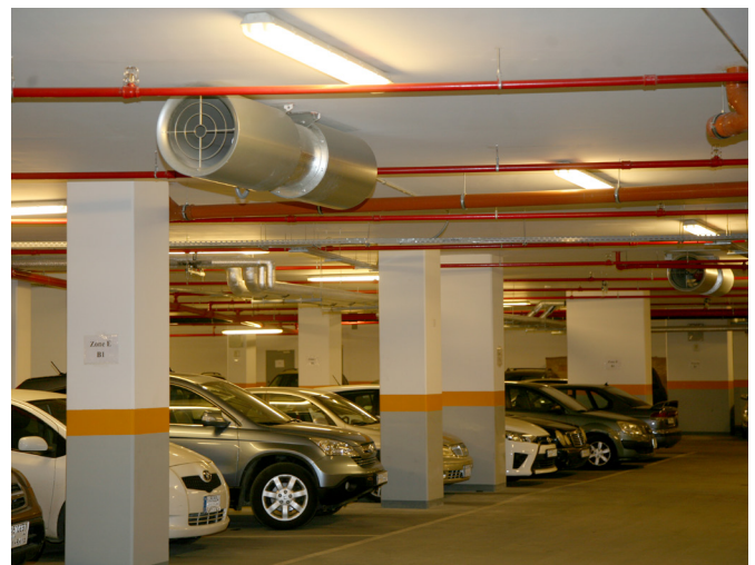
Fig. 4(c): Systemair 400-2-(B) TR Jet Fans
