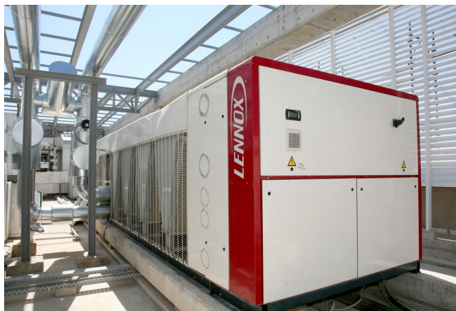
Fig. 2(a): Lennox NEOSYS NAC 960F NM4M
