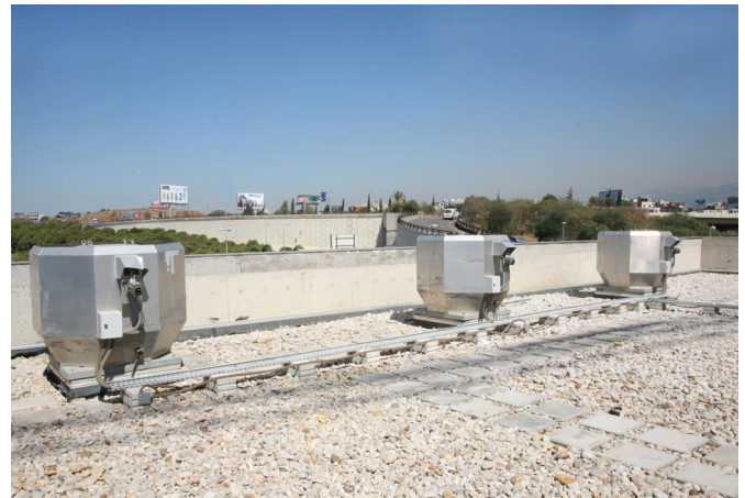
Fig. 5(b): 3 No. Systemair Smoke Extract Fan DW 1000 D4-F400 for Cock-Pit Simulator Area
