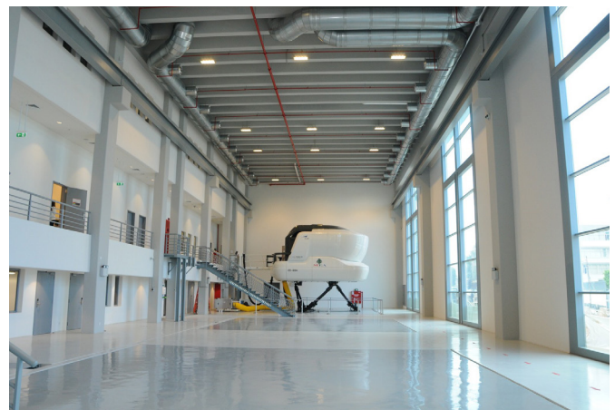
Fig. 5(c): Systemair Jet Diffusers AJD-400
